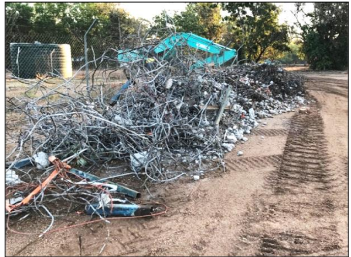
Photo 6. Steel extracted from crushed concrete
