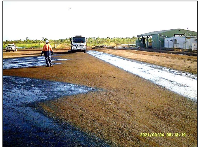
Photo 11. First prime to place recycled Asphalt
