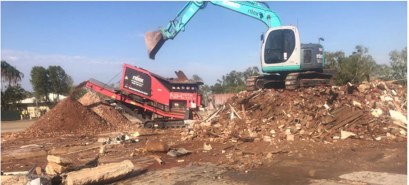
Photo 2. Hammbreaker Crusher in action at Katherine Sports Club demolition
