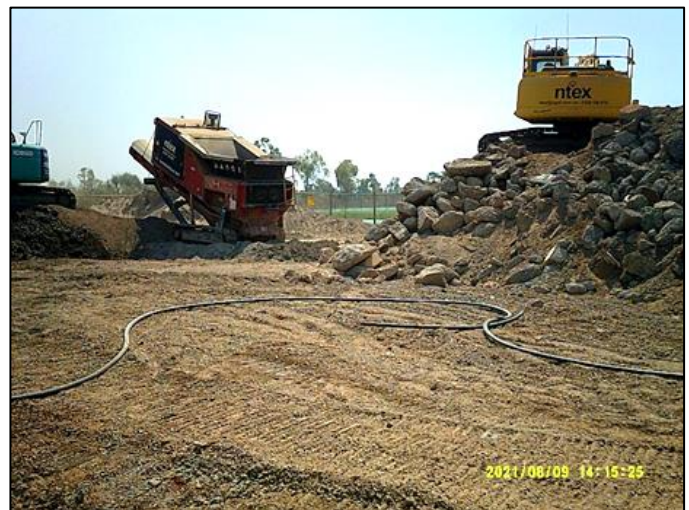
Photo 9. Crushing concrete
