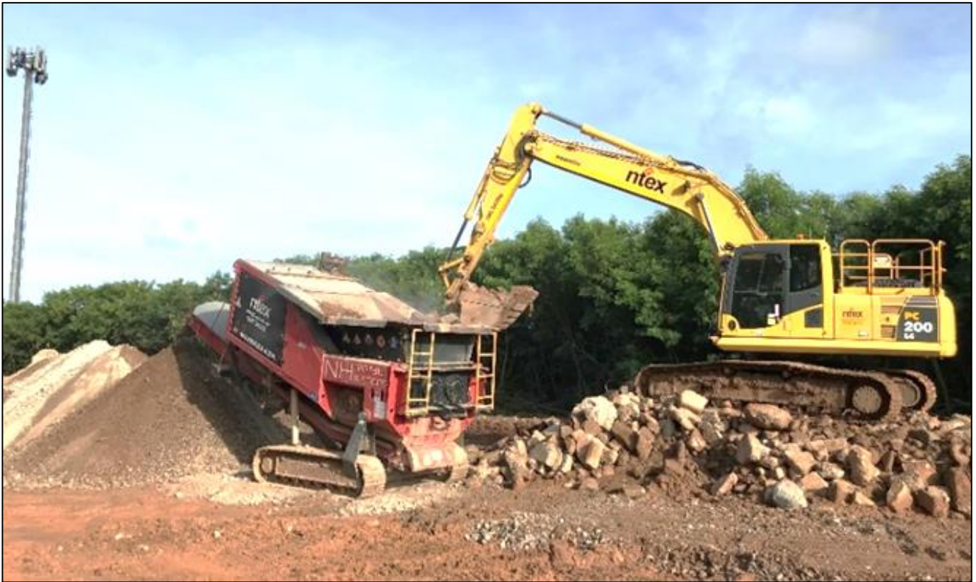
Photo 4. Feeding concrete into crushing unit
