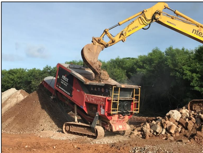
Photo 19. Concrete crushing
